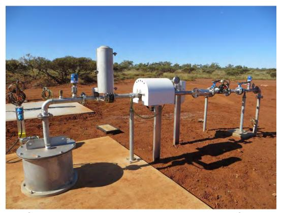
Figure C4 New electrically powered production bore within the Cane River Water Reserve, photograph by V. Claughton, Department of Water
