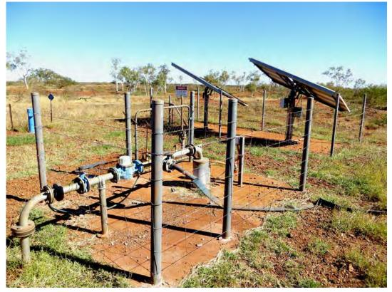
Figure C6 A solar powered production bore within the Cane River Water Reserve, photograph by V. Claughton, Department of Water
