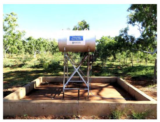
Figure C5 A bunded fuel tank used to power a production bore within the Cane River Water Reserve, photograph by V. Claughton, Department of Water
