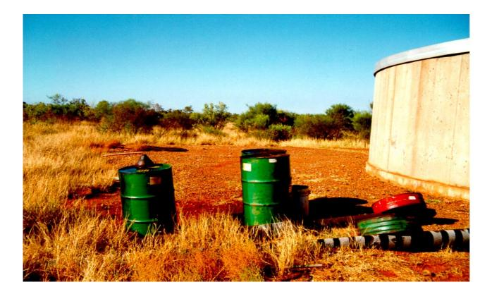
Plate 3. Unbunded oil drum storage at the pumping station
