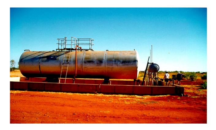
Plate 2. Bulk diesel storage at the pumping station
