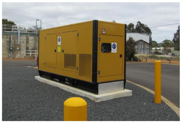
Figure D5 Self-bunded diesel generator
