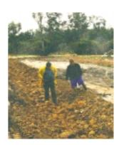
Rocked chute under construction on an eroding sandy gully, Manjimup.
