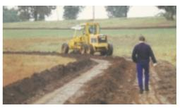
Permanent grade banks – planned, surveyed and shown being constructed by a road grader.
