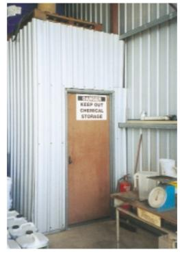
This chemical shed is well marked, but it should have been located away from other buildings and the chemicals should be locked inside it at all times.
