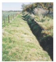
A fenced buffer strip reduces nutrient export into the drain and protects vegetation.
