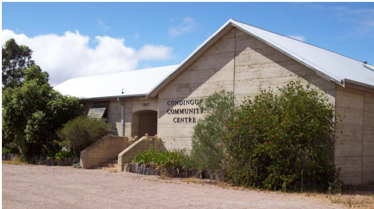
Photo 3 Condingup Community Centre
