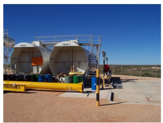
Figure D6 Diesel storage tanks (externally bunded) at the Coral Bay power station [Photo: B. Franke]
