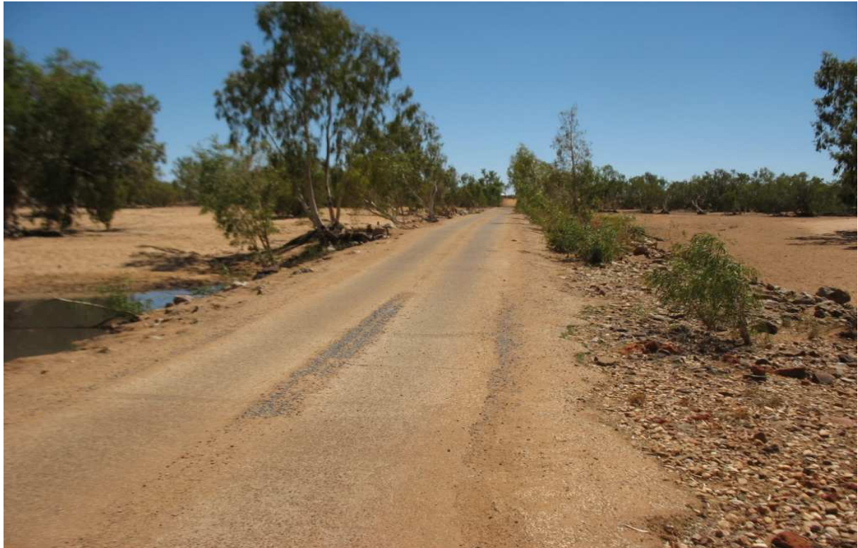
Photo 1 – Gascoyne River crossing
