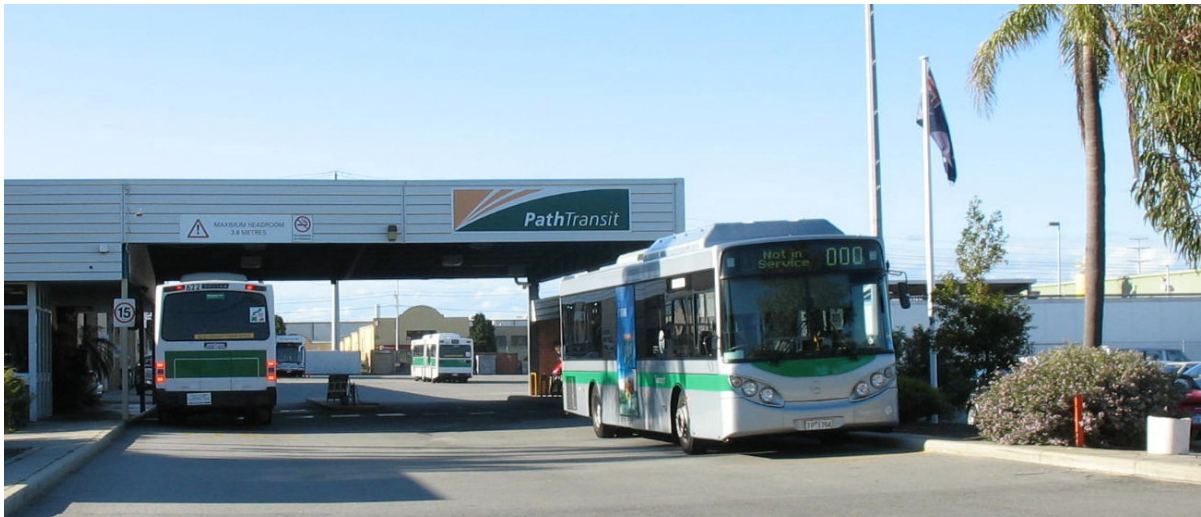
Photo. 4 Path Transit bus depot – Malaga Industrial Area Industrial Zone Precinct 69
