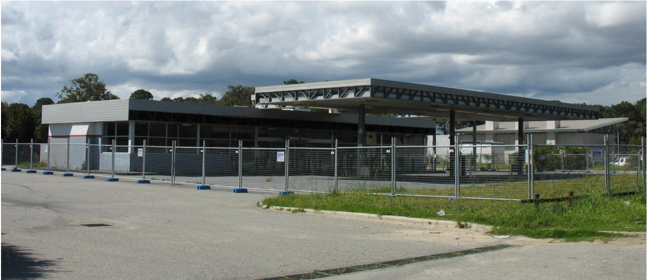
Photo. 13 Abandoned Petrol Station – Gngangara Rd Special Rural P1 Area - Lexia Rural Zone Precinct 54
