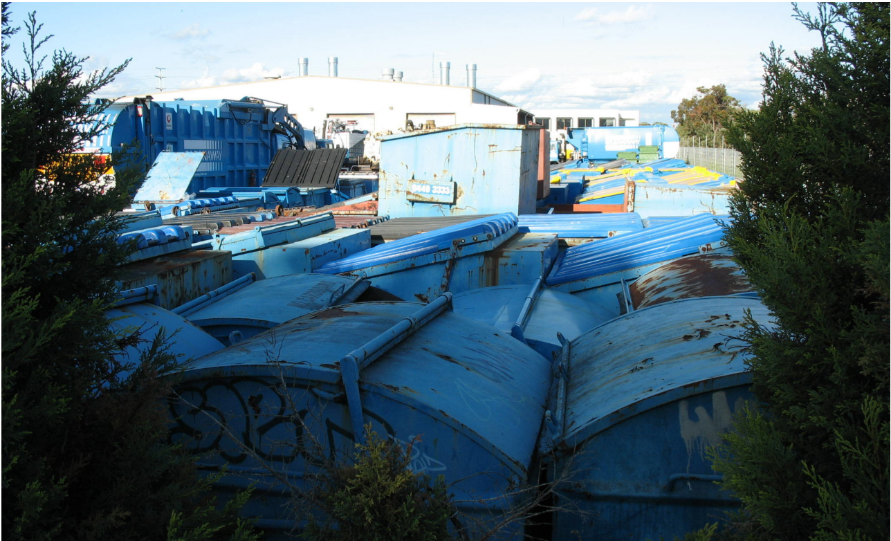
Photo. 3 Waste depot – Malaga Industrial Area Industrial Zone Precinct 69
