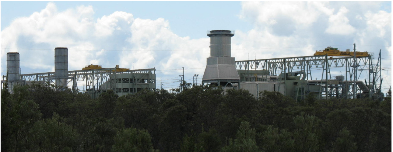
Photo. 21 Western Power Pinjar Power Station - Pinjar Public Purpose Reservation Precinct 32
