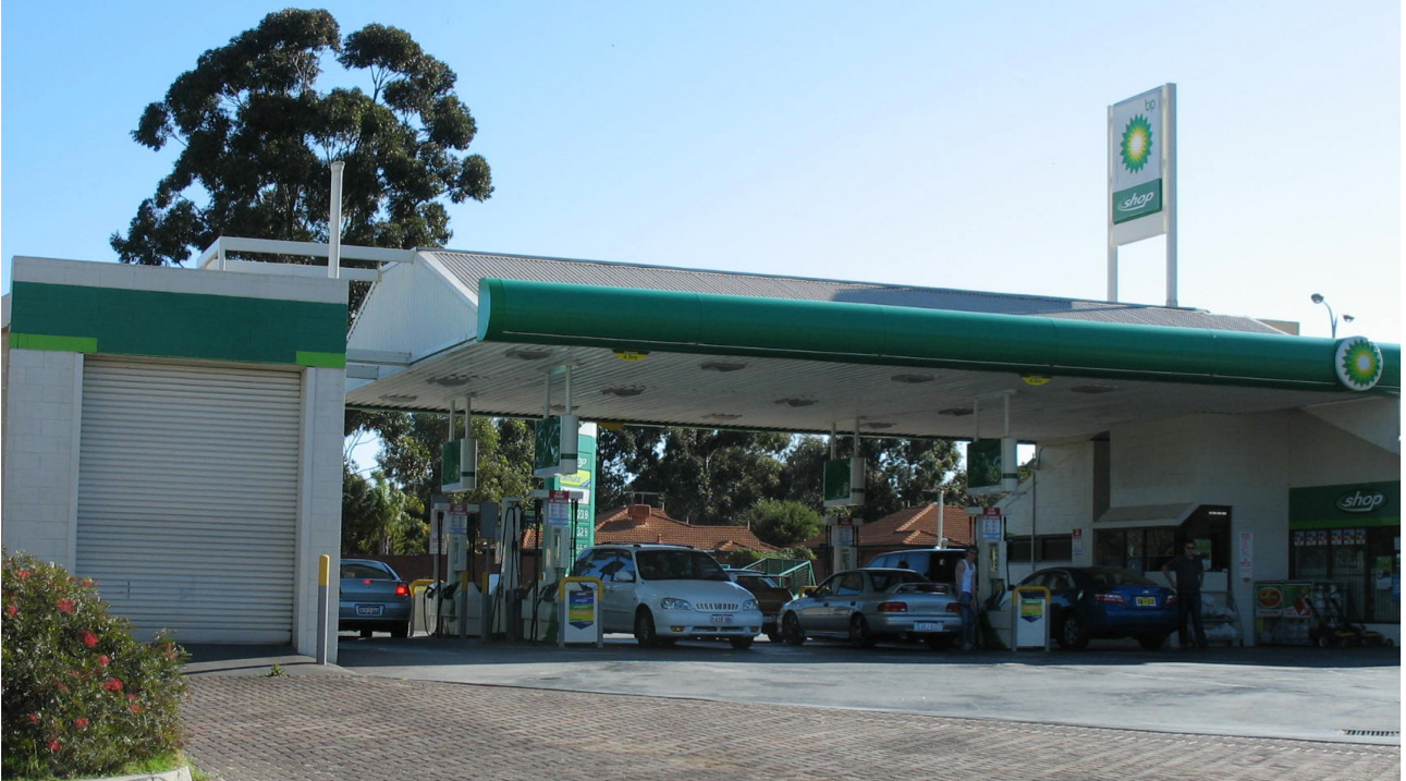
Photo. 11 Petrol Station - Ballajura Urban Zone Precinct 69
