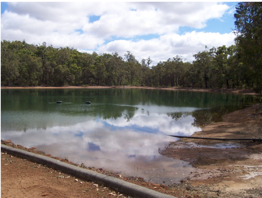
Figure D2 Exposed reservoir banks at Hester Dam, photograph by B. Franke 2008
