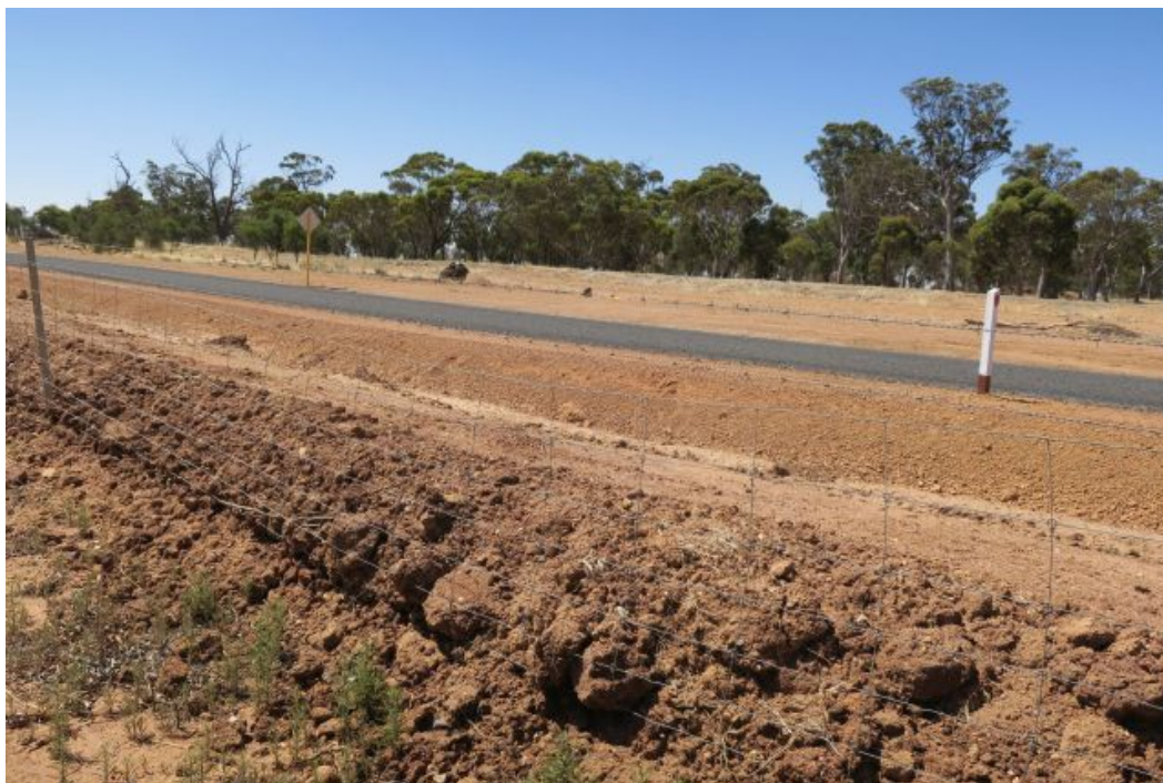
Figure C8 Katanning Catchment Area fencing and neighbouring road and railway
