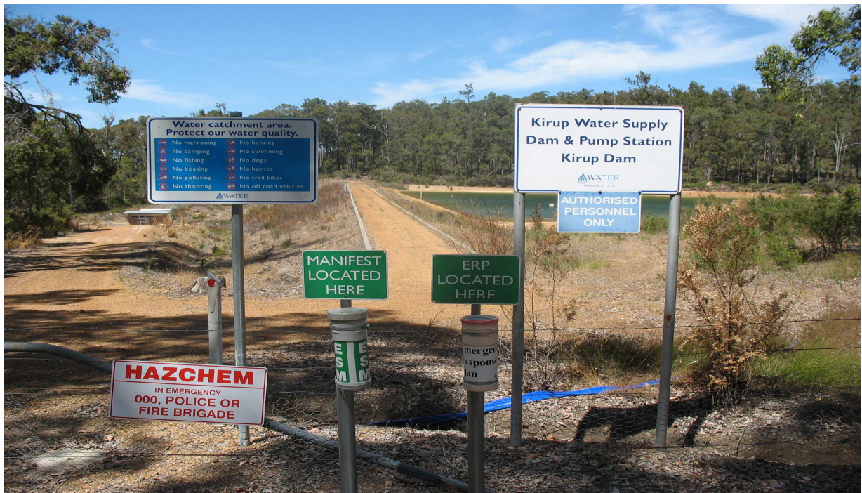
Photo 3 Kirup dam signage to reservoir fence. December 2006
