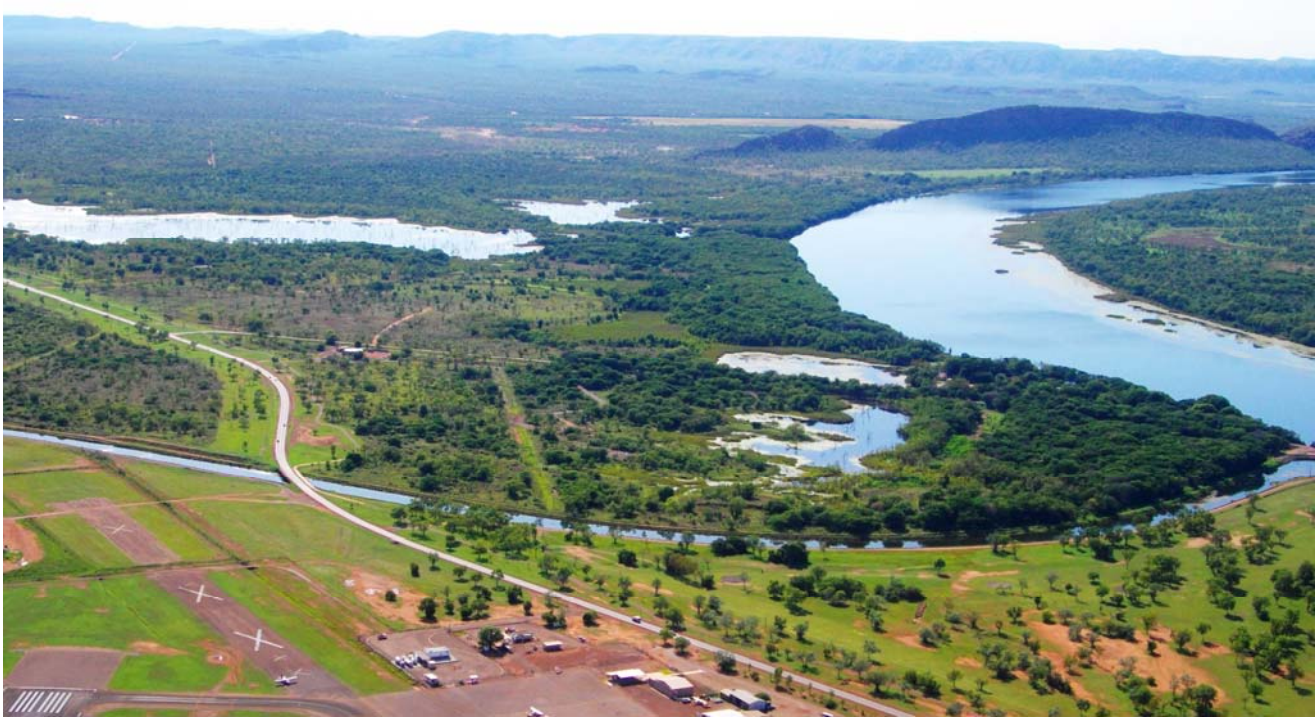
Figure D1 Kununurra Water Reserve as viewed from the north-west. The M1 channel visible in the foreground is next to the western boundary of the water reserve. Lily Creek Lagoon in the background forms part of the eastern boundary. The Kununurra Airport and golf course in the foreground are not within the water reserve boundary. (Photographer: Stephen Watson)
