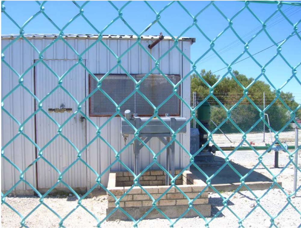
Figure C3 Production bore 1/81 – diesel standby bore, photograph by J. King, Department of Water
