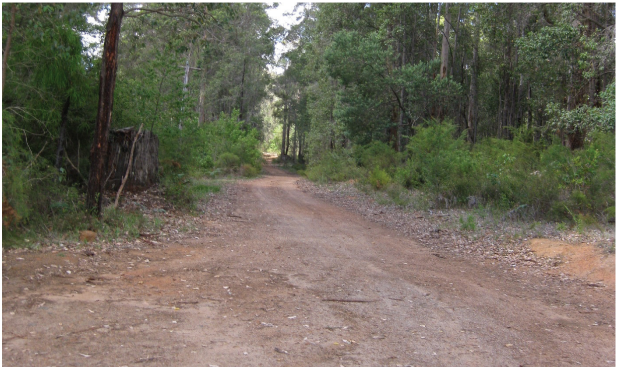
Figure D4 Unsealed road within the Phillips Creek Dam Catchment Area
