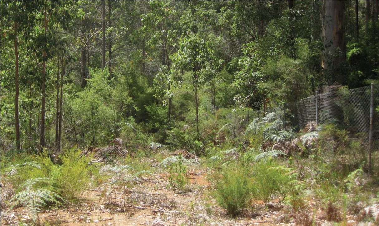
Figure D6 Fence limiting access to the Phillips Creek Dam
