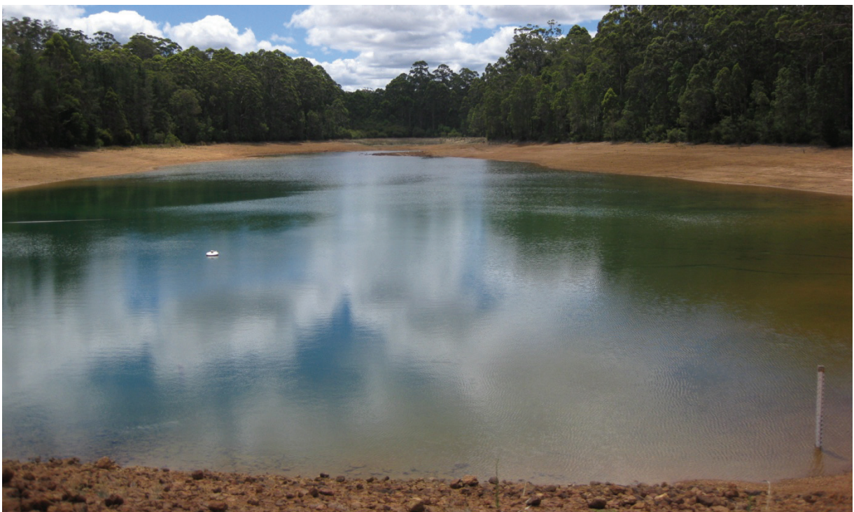
Figure D2 Phillips Creek Dam Reservoir
