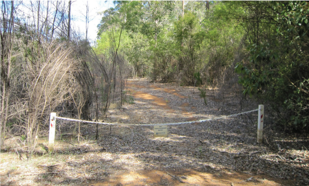
Figure D5 Chain gate limiting access to the Manjimup Dam
