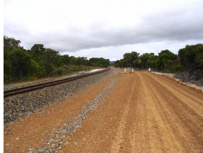
Photo 6 Railway line and access track adjacent to Brook
