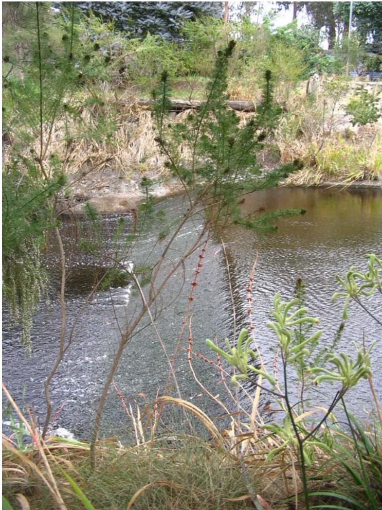
Photo 1 Gauging station weir at Elleker Bridge
