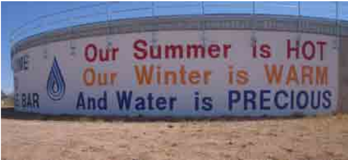
Figure D1 Water storage tank Marble Bar
