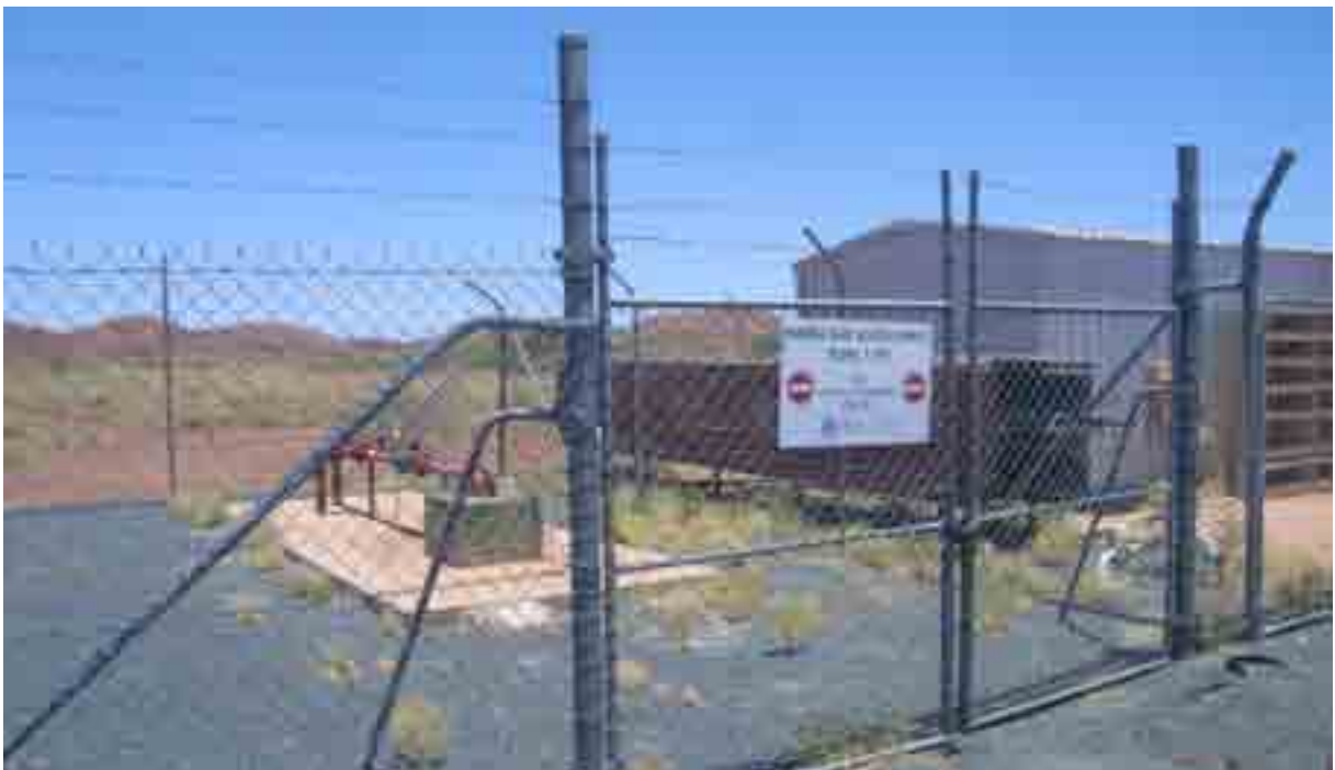
Figure D4 Production bore 1/99 and associated storage and maintenance shed in the Coongan wellfield
