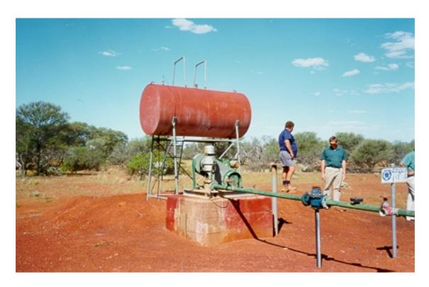
Plate 2. Production bore 5/85 and elevated fuel storage tank. Similar to production bore 12/85.
