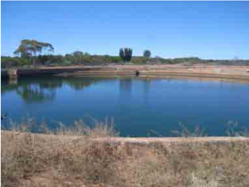
Figure D3 Menzies Town Dam No. 1
