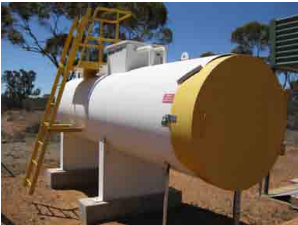
Figure D2 Self-bunded diesel wrap tank
