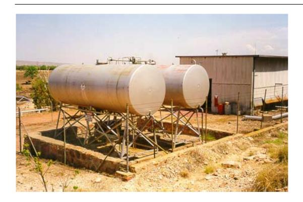
Plate 3. Bunding arrangements for diesel storage at the Moochalabra Pump Station. Bunding is inadequate to capture 'jetting' leaks.
