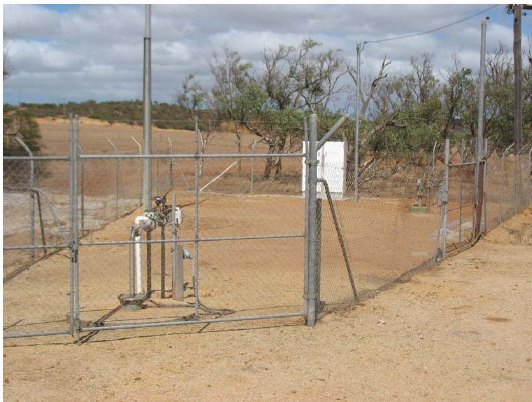
Photograph 2 Water Corporation bores 5/94 and 10/83 in a locked compound
