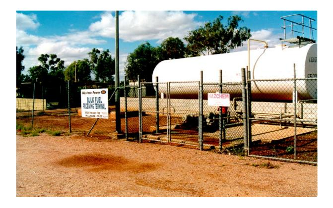
Plate 3. Diesel fuel storage at the Western Power Station
