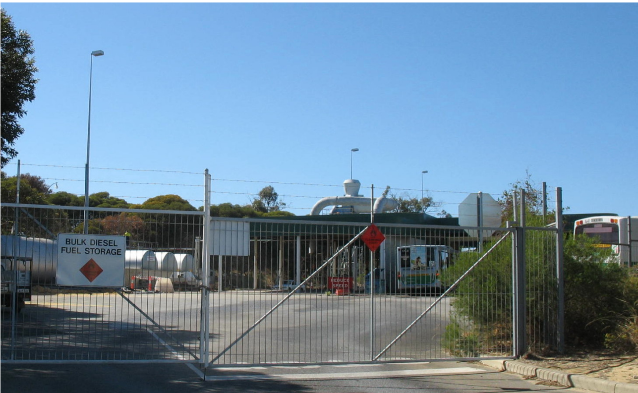
Photo. 13 Path Transit bus depot – contaminated site – Joondalup Urban Zone Precinct No 49
