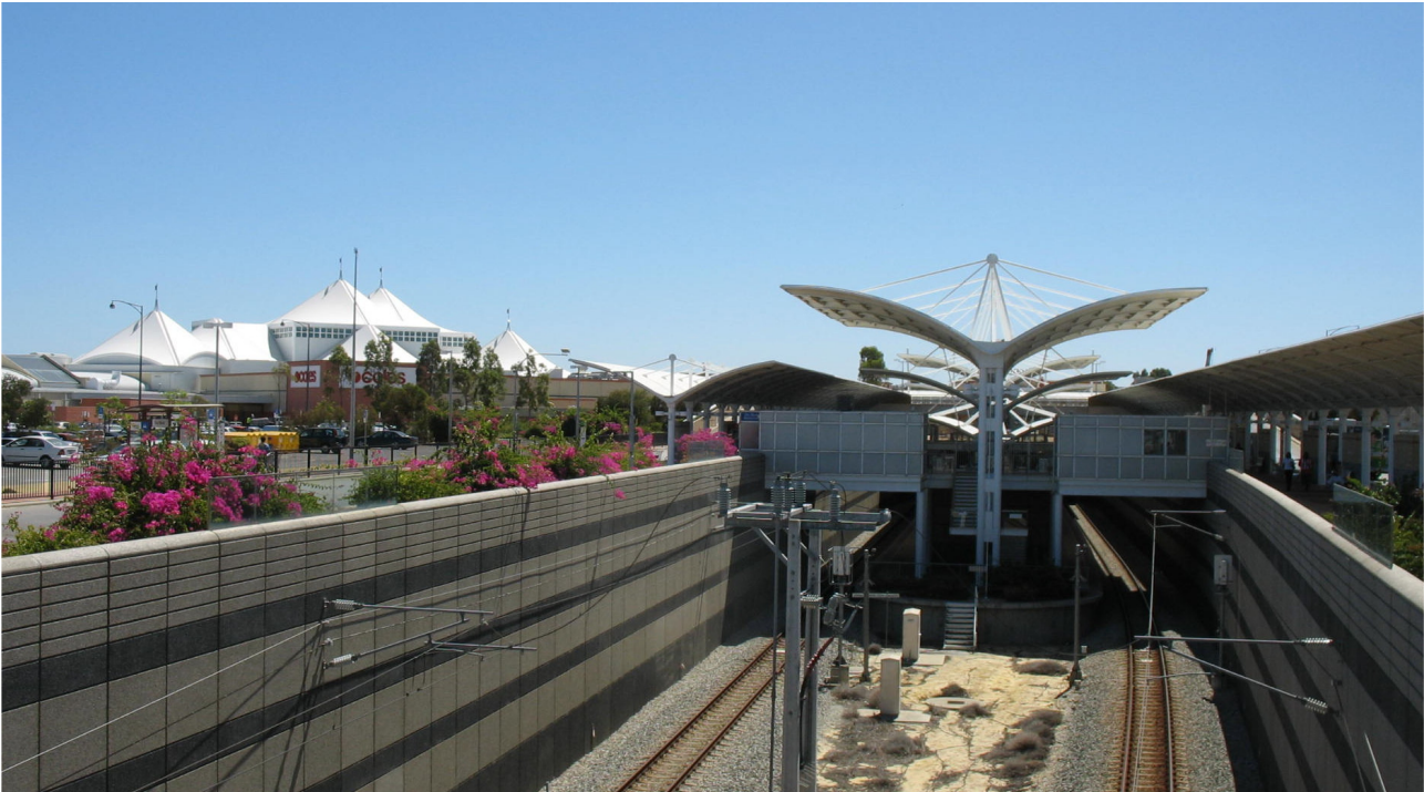
Photo. 24 Metrorail – Joondalup Station Central City Zone Precinct No 50
