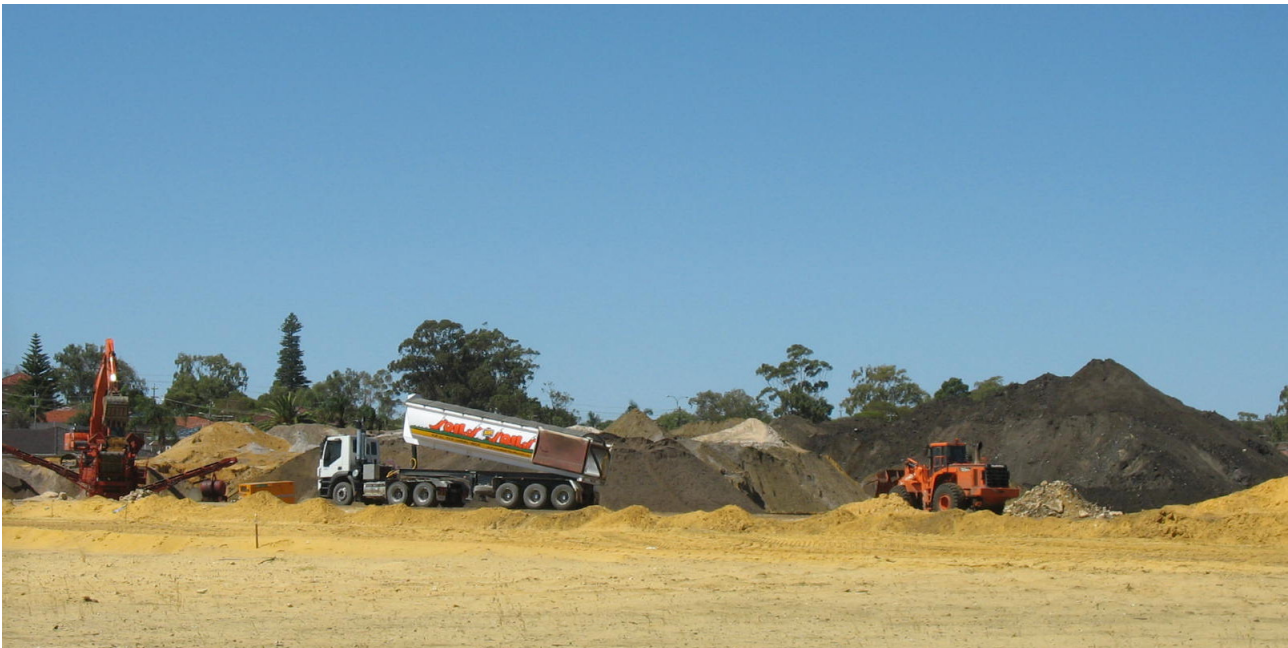
Photo. 18 Peat excavation at Roselea Estate - Stirling Urban Zone Precinct No 92
