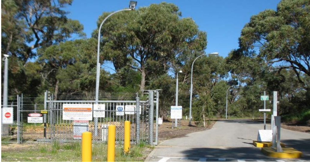
Figure C3 Entrance to Neerabup groundwater treatment plant
