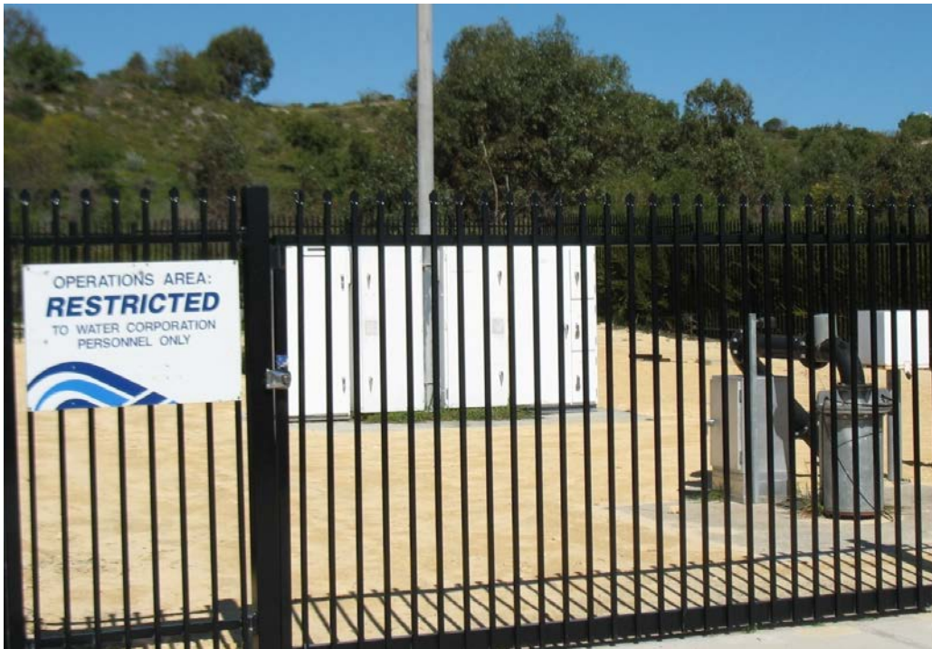
Figure C1 Water Corporation compound at Kalbarri Avenue, Yanchep
