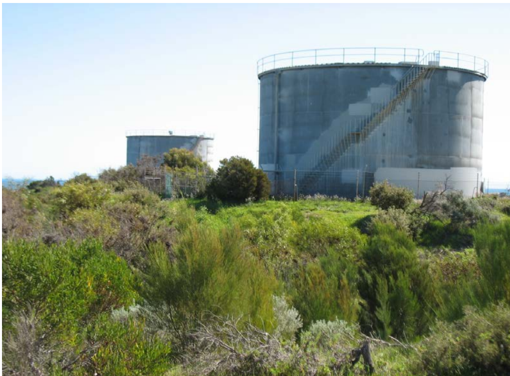
Figure C2 Yanchep drinking water storage tanks
