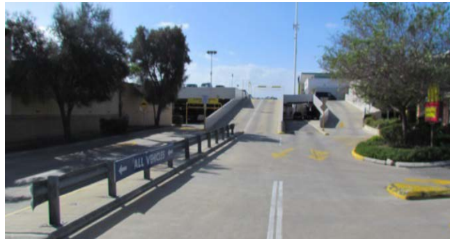
Figure 14. Ramp from Rockingham Road
