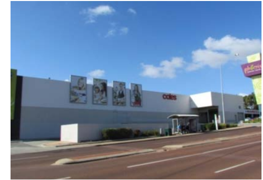
Figure 20. Rockingham Road servicing area
