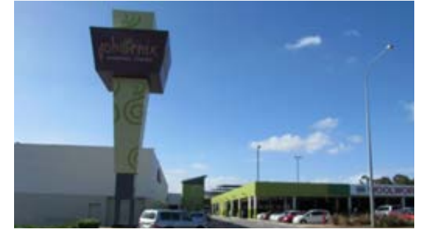
Figure 18. Southern entrance from Rockingham Road, currently relies on signage, proposed relocation south
