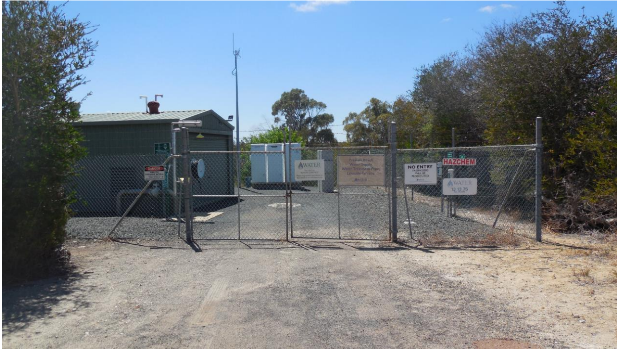
Figure C3 The entrance to bore 2/85 and Preston Beach's drinking water treatment plant is securely fenced and signed
