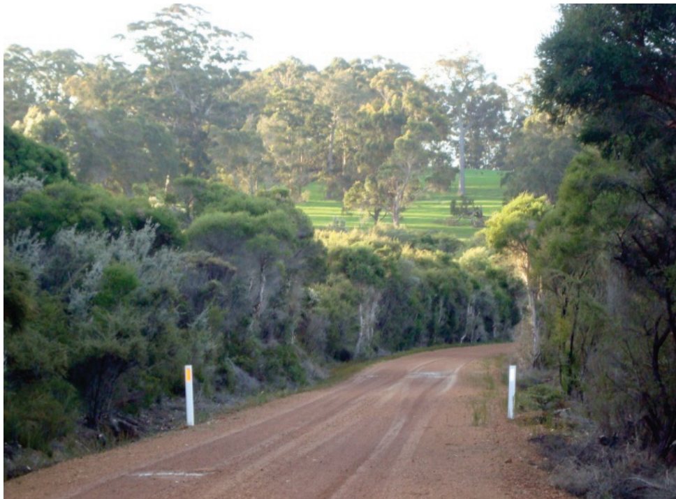
Figure D3 Access way to Quickup dam (public access prevented by locked gate).
