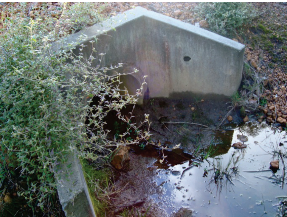
Figure D2 Culvert
