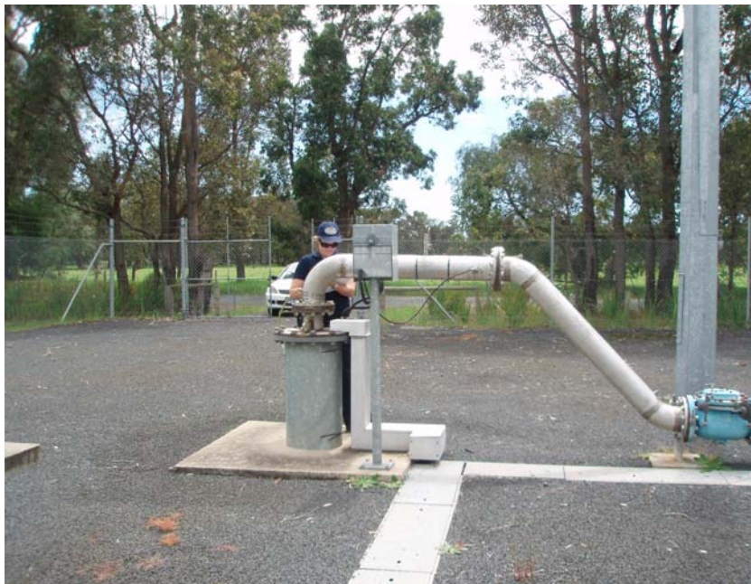
Photo 2 Bore 3/98 sourced from the Sue Coal Measures
