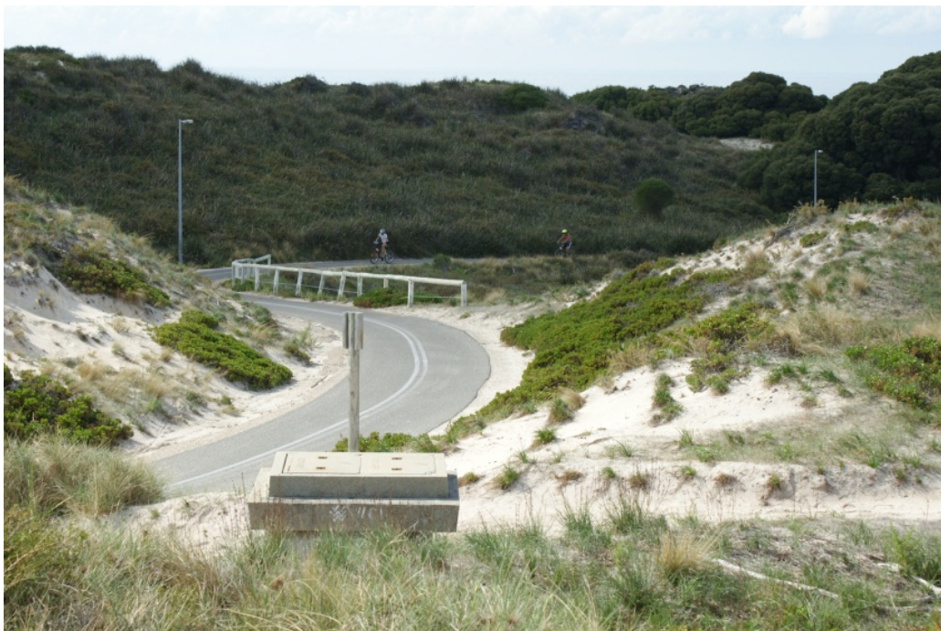
Figure C12 Vents for sewer pump stations and sealed roads in Longreach Bay saltwater bore field, photograph by C. Loos
