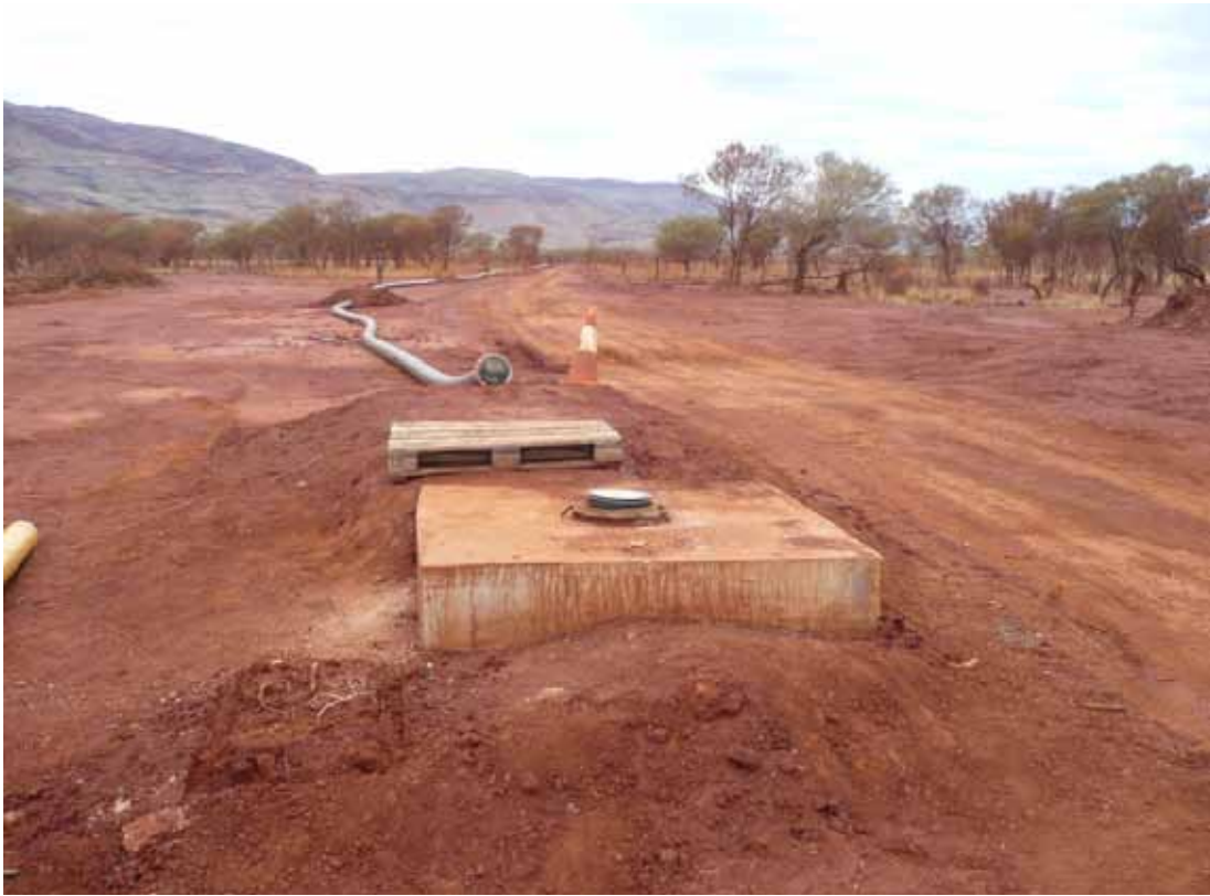
Figure D7 Southern Fortescue reinjection bore
