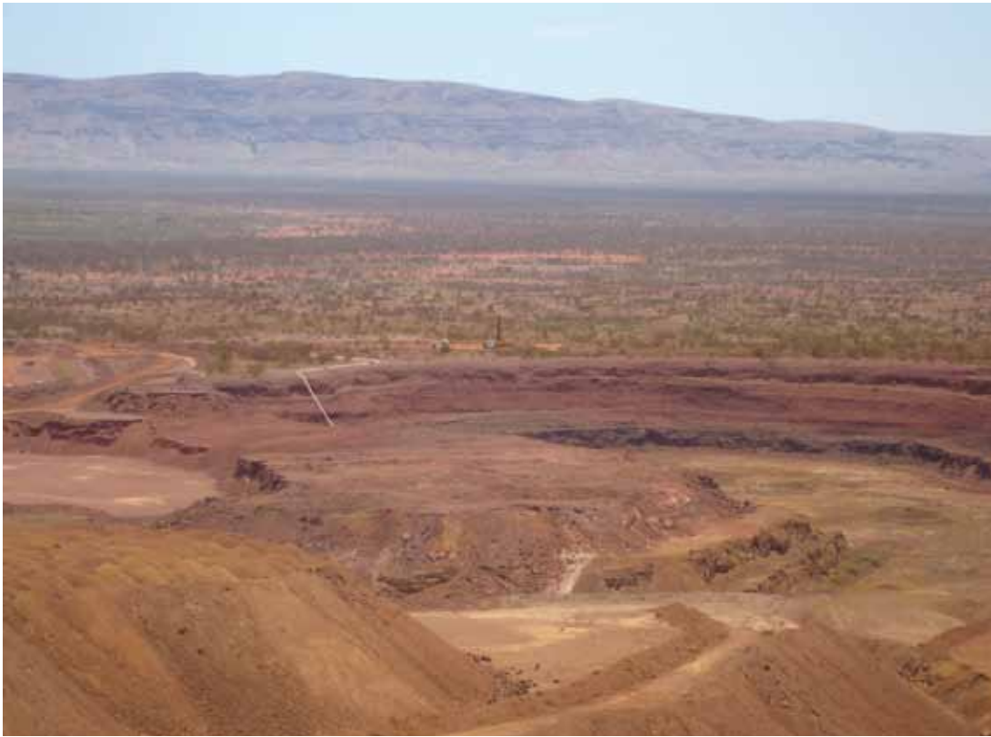
Figure D3 Drilling dewatering bores at Marandoo
