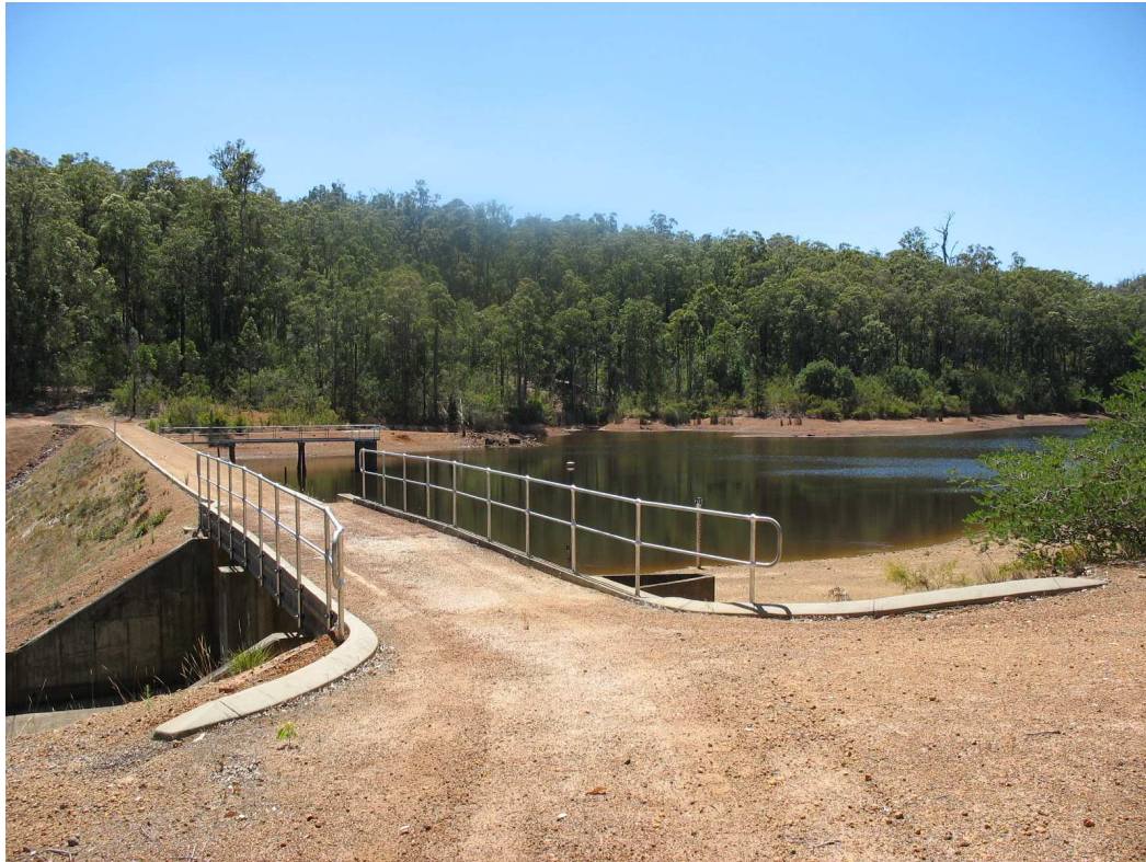
Photograph 1 Tanjannerup Creek Dam
