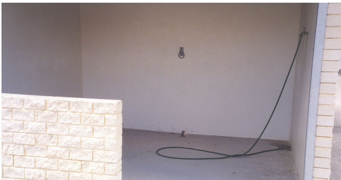
Roofed wash-down bay with drainage
