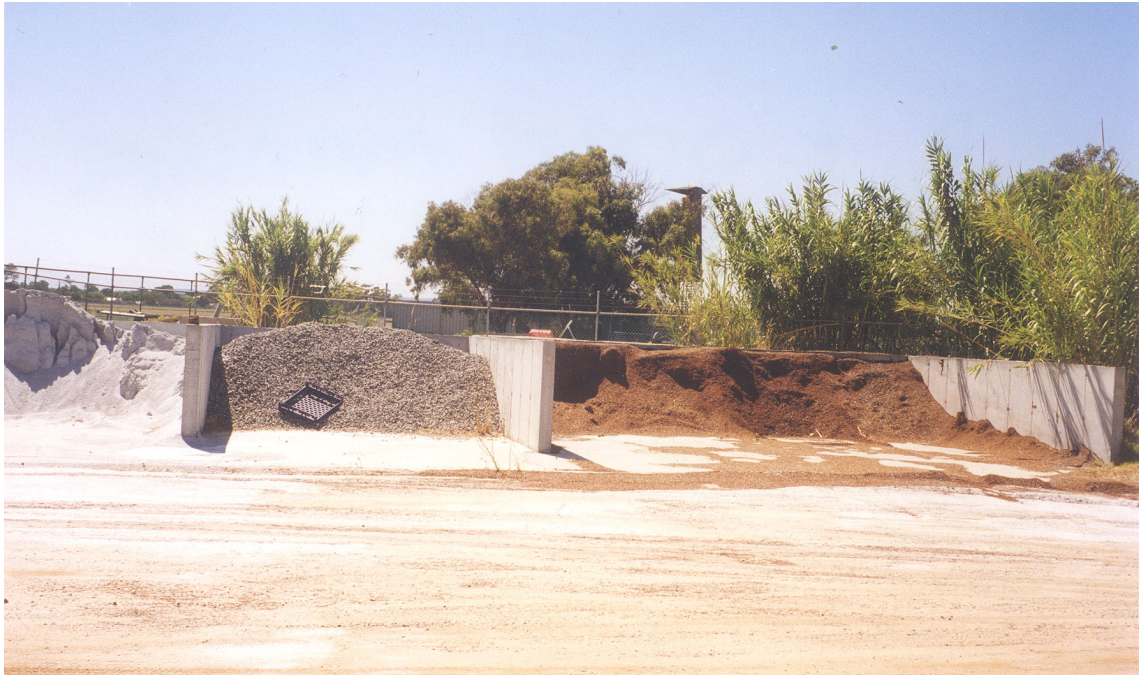
Contained storage of woodchips and manure on an impermeable surface
