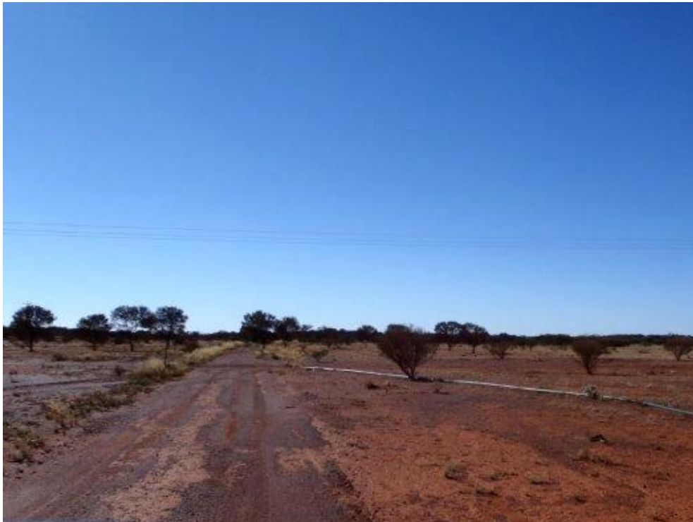
Figure C7 Unsealed road within the Wiluna Water Reserve, photograph by M. Sawyer, Water Corporation, reproduced with permission
