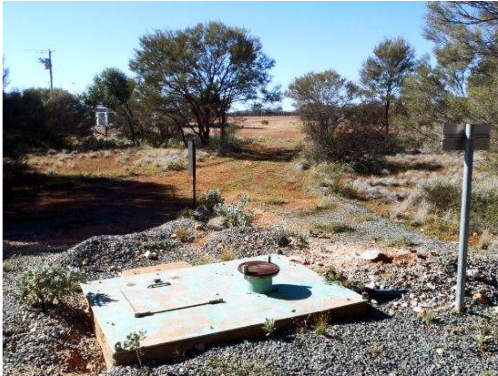
Figure C5 A decommissioned bore within the Wiluna Water Reserve, photograph by M. Sawyer, Water Corporation, reproduced with permission
