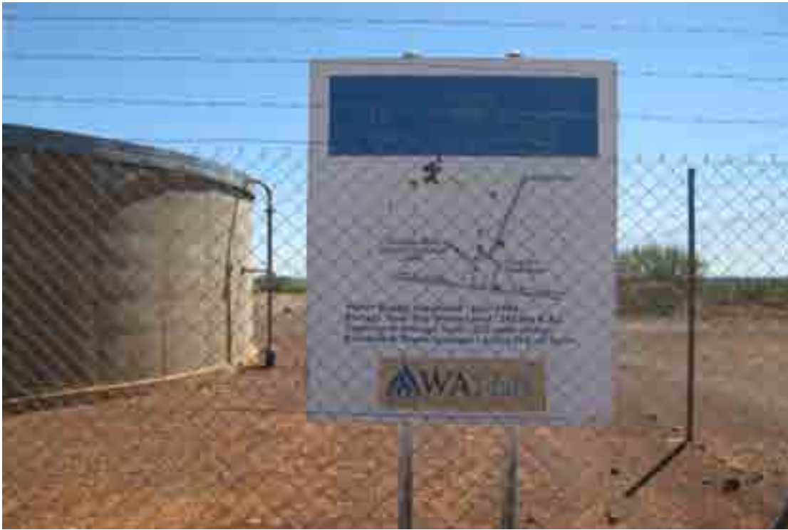
Photo 3 Groundwater is abstracted from the Yalgoo Borefield before being treated, pumped to the Yalgoo storage tank (where photo taken) and gravity fed into Yalgoo town.
