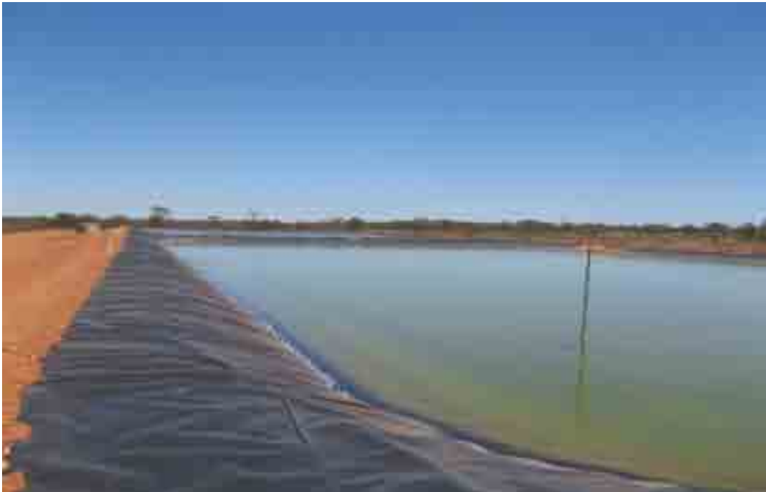
Photo 5 Evaporation ponds, located across the road from the Yalgoo drinking water treatment plant, store & evaporate wastewater from the plant.
