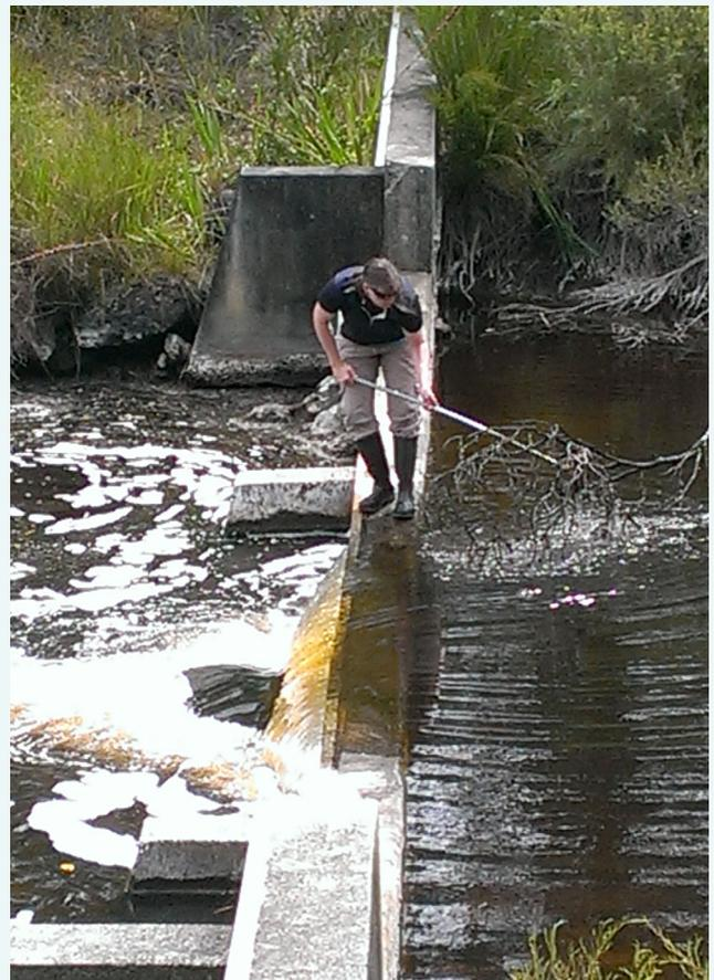
Cleaning debris off the weir at the Kalgan River sampling site. High flows can wash debris onto the weir, which impacts flow measurements, November 2015.
