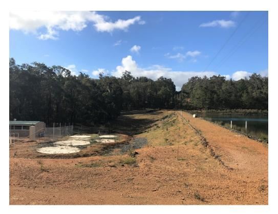
Figure C4 Dumpling Gully Dam 1 showing decommissioned water supply tanks due to the source being no longer used by the Water Corporation
