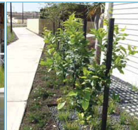
On-lot biofilter, Evermore Heights, Baldivis
