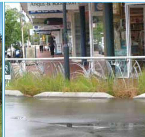
Roadside biofilter retrofit, Busselton CBD
