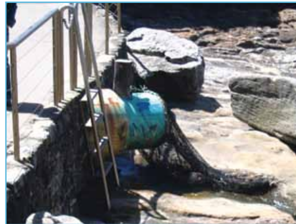
Release nets – netting installed on pipe outlets to collect litter
