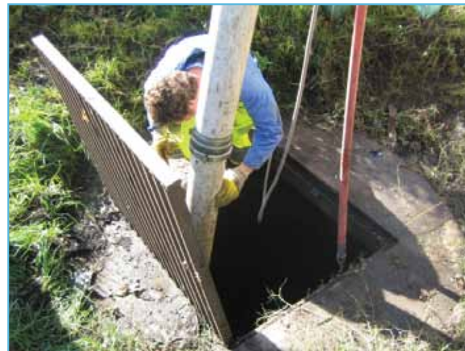
Gross pollutant traps require regular maintenance
