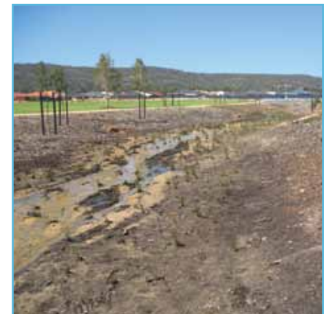
Newly constructed living stream, Byford
