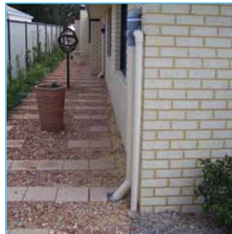
Pervious aggregate placed around impervious pavers
