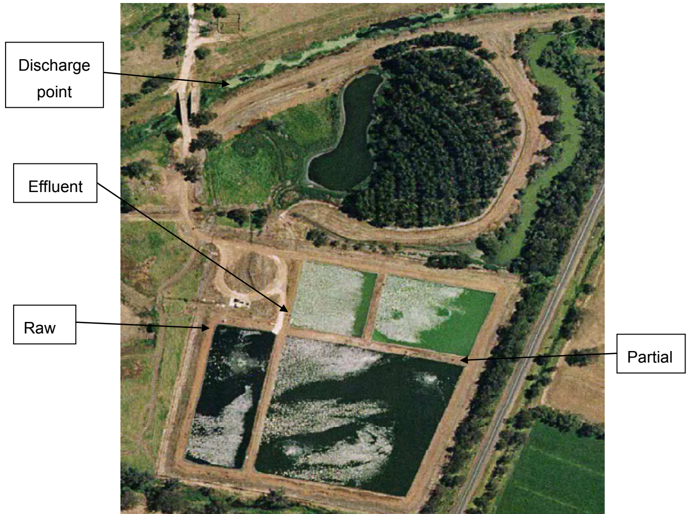
Figure 7: Annotated aerial photograph of Harvey WWTP
