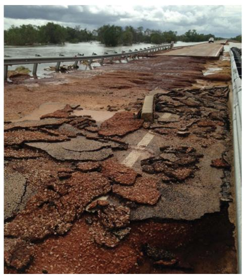
Figure 35. Flood damage to the Logue River bridge in the Kimberley. Source: Main Roads WA
