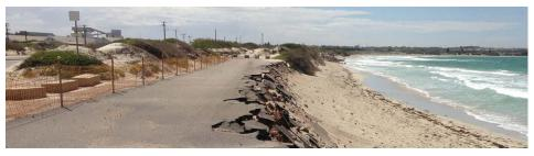
Figure 15. Coastal erosion in Geraldton. Source: Department of Transport
