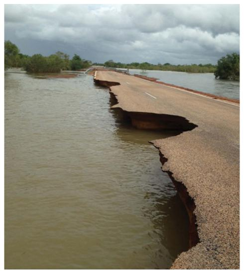
Figure 36. Flood damage near the Logue River bridge in the Kimberley. Source: Main Roads WA
