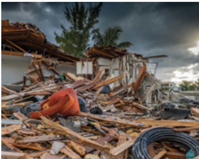
Clean-up work of affected properties after Hurricane Katrina
