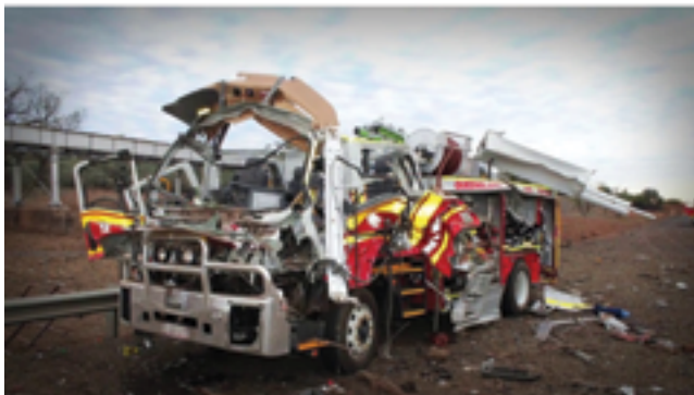
Top: Complete destruction of the Angellala Creek road bridge. Bottom: Damage to fire trucks as a result of the explosion
