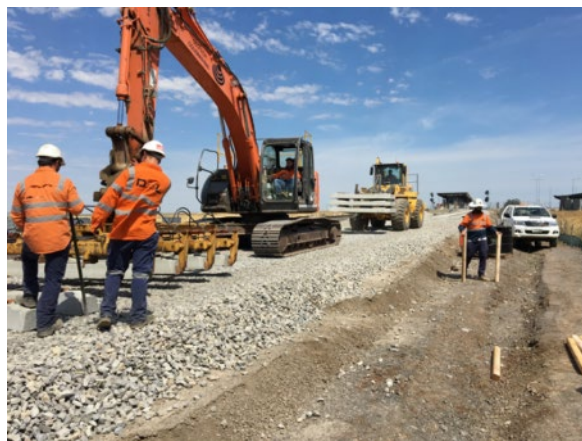
FIGURE 165: SLEEPER PLACEMENT USING OCTOPUS GRAB
