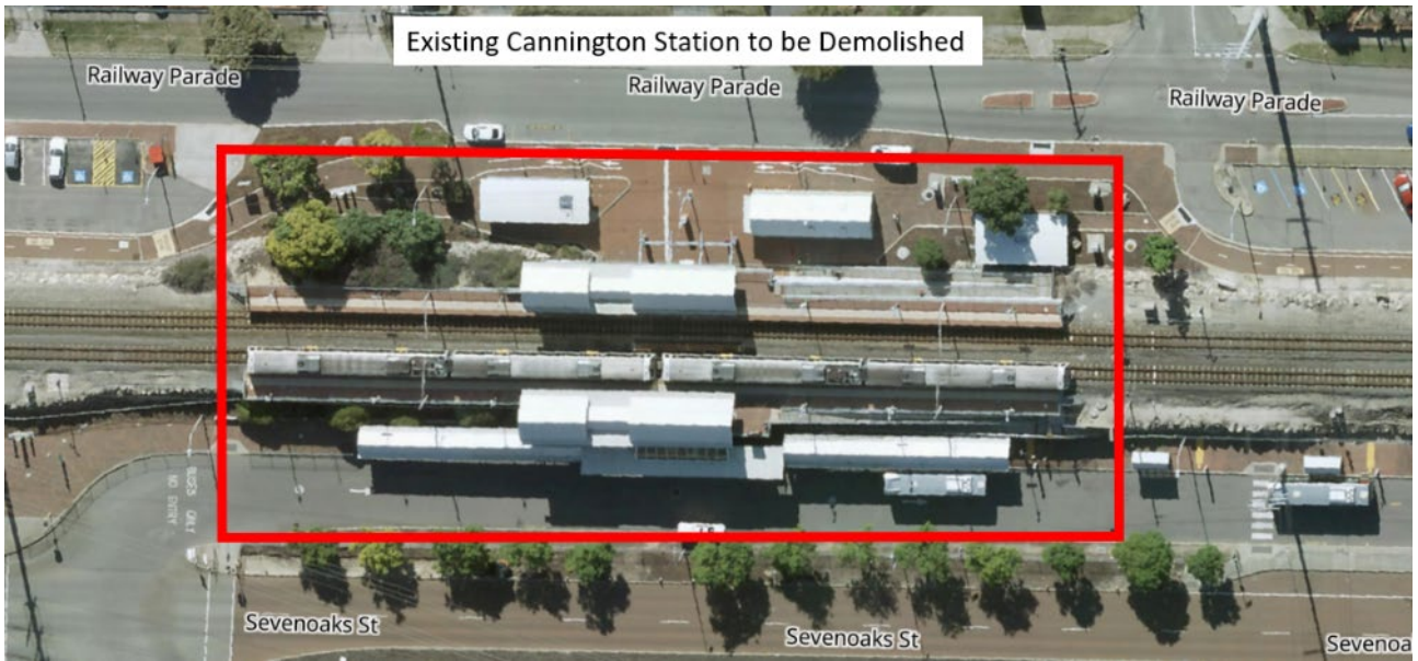
FIGURE 125: CANNINGTON STATION TO BE DEMOLISHED (CARPARK DEMOLITION COVERED IN CIVIL SCOPE)
