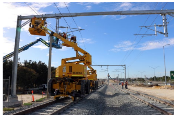
FIGURE 171: OLE MAST INSTALLATION - VIADUCT
