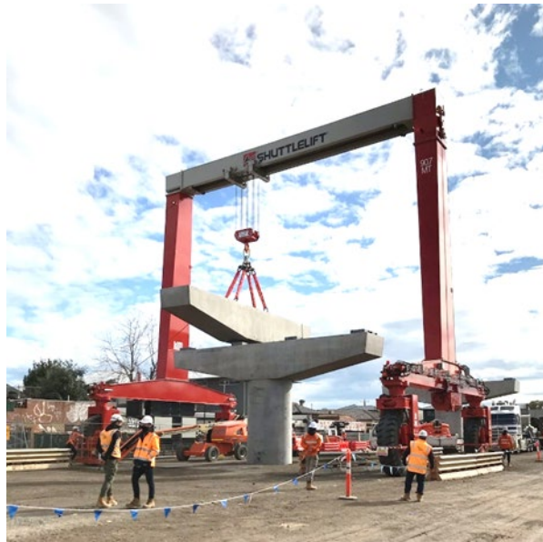
Dual Crane Crosshead lifts
