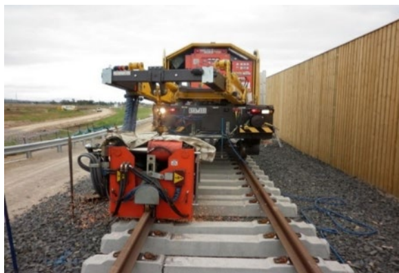
FIGURE 163: MOBILE (HIRAIL) FLASHBUTT WELDER IN OPERATION
