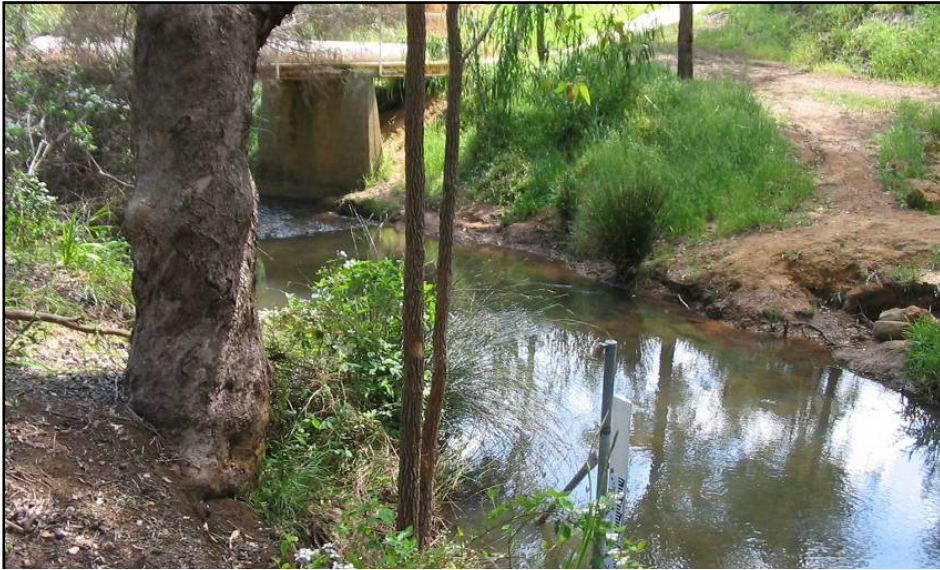
Figure 11 View of Reach 3 (Bernard Street) near the control point
