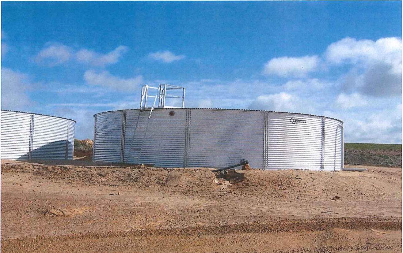
Figure 3. Storage tanks, King Rocks Community Dam, Kondinin Shire
