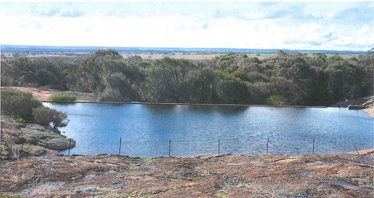
Figure 1. McGanns Rock Dam, Kondinin Shire
