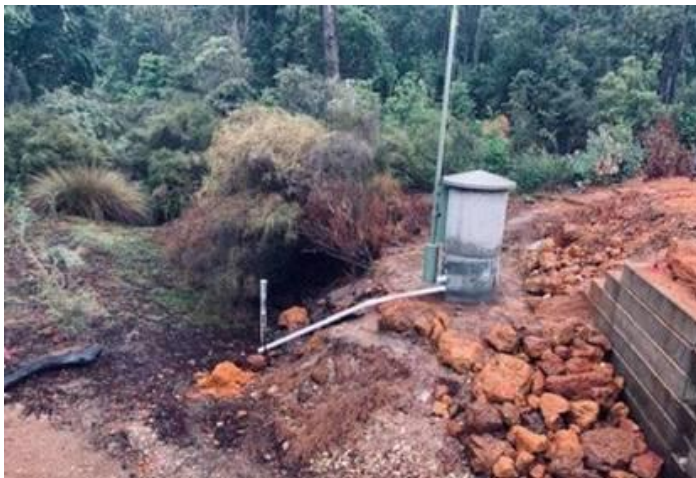
Above – Temporary floatwell installation completed 9 April 2020 at Manjimup Brook outflow
