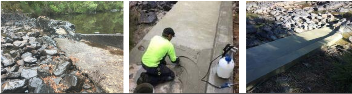
Above – Strickland Gauging station before (left), during (center) and after (right) remedial works had been completed to repair cracking, undercutting and wear.
