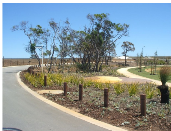
Photo 19: Flush kerbing to allow frequent stormwater events to flow to vegetated areas for treatment and infiltration, retaining natural bush where possible. Public open space, Seascapes, Halls Head.
