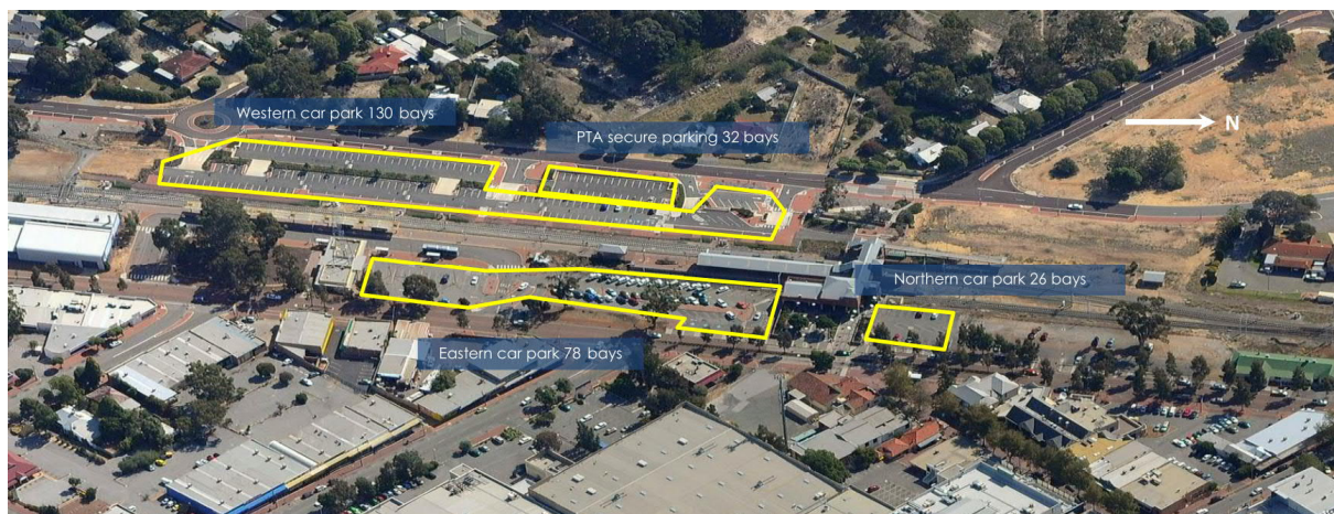
Figure 5 Aerial view of the PnR facilities at Armadale Station (PTA)
