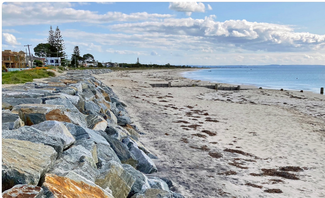
Granite seawall, Busselton – Photo courtesy WALGA
