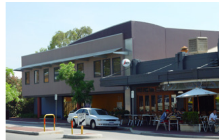
High Street Station
